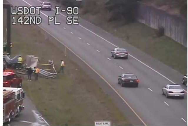
Figure 1-6: Cabinet damage due to guardrail deflection
